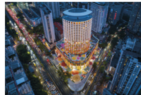
SHENZHEN WOMEN & CHILDREN'S CENTER Shenzhen, China Architect: MVRDV Developer: Shum Yip Group Limited Others: Façade consultant: KGE (King Glass Engineering); Structural Engineer: Yuanlizhu Engineering Consultants; Lighting Consultant: BPI (Brandston Partnership Inc.); Cost Calculation: Jinxia Property Cost Consultation Co. Ltd.; Interior Architect: Jiang & Associates
