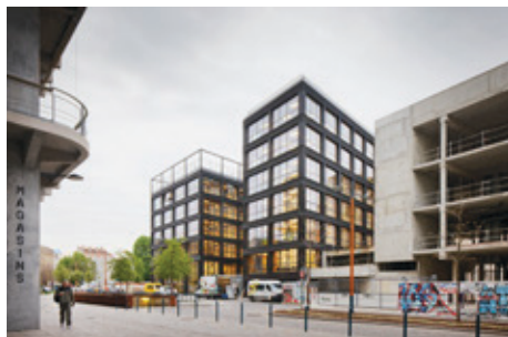
WoodE Pantin, France Architect: Chartier Dalix Developer: PRD OFFICE
