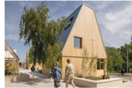
Living Places Copenhagen Copenhagen, Denmark Developer: VELUX Architect: EFFEKT Others: Artelia, Enemærke & Petersen
