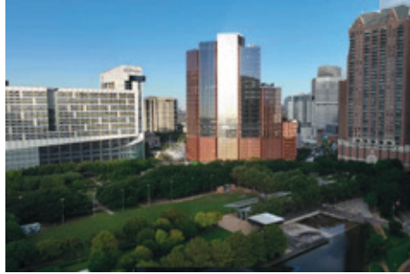
1550 on the Green Houston - Texas, United States Architect: Bjarke Ingels Group (BIG) Developer: Skanska USA Commercial Development
