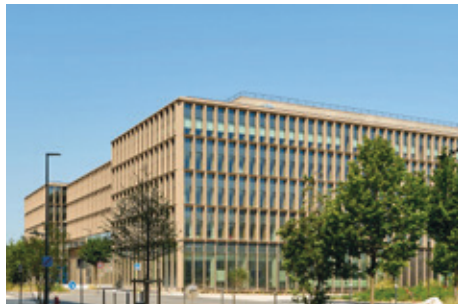
International Center of Research and Innovation Daniel Carasso of Danone Plateau de Saclay (Gif-sur-Yvette), France Architect: Arte Charpentier Developer: Danone Other: Eiffage
