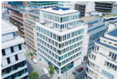
Monteco Brussels, Belgium Architect: ARCHi2000 Developer: ION and Nextensa
